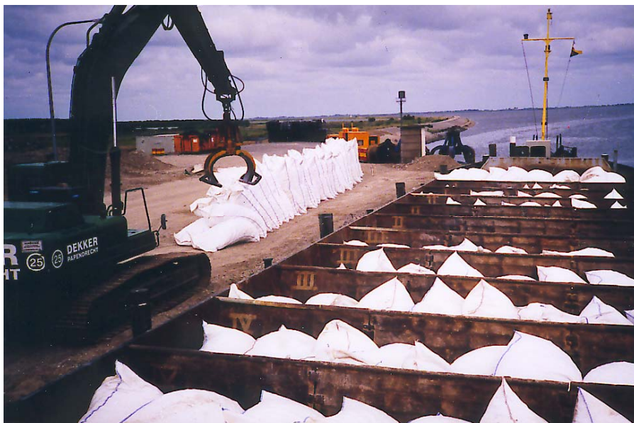
Figure 2 : Filling and loading of sand bags at Eider Storm Surge Barrier, Germany
