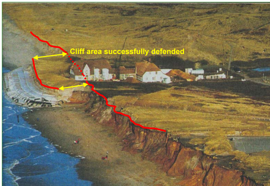
Figure 1 : Defended cliff area with geotextile “sand cushions” on the Island of Sylt, Germany
