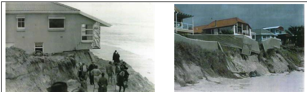
Photos 1 & 2; Typical Erosion, 1967 and 2000
