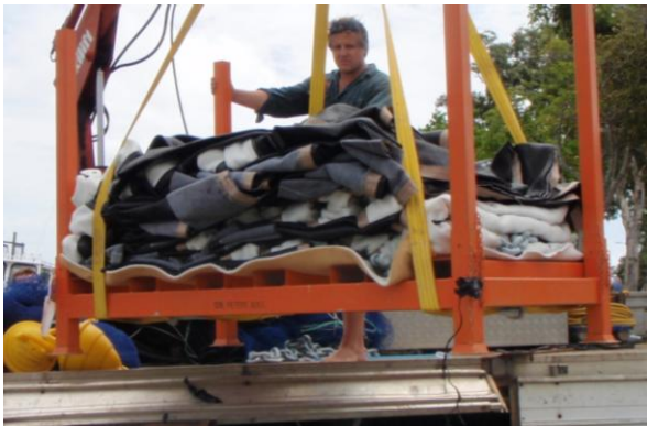
Figure 15: Seabed-based algae curtain prior to installation
