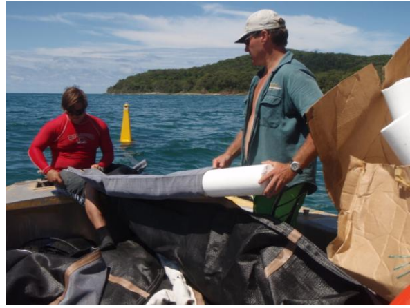
Figure 16: Final assembly and deployment of algae curtain
